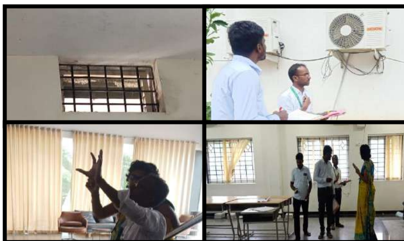
Ventilation and Exhaust system Facilities in SAWC Buildings
